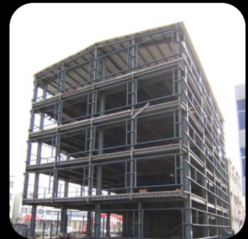
Multistory Steel Building
