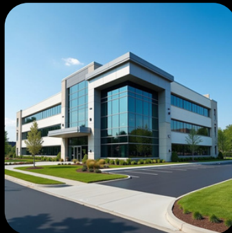
Office building construction
