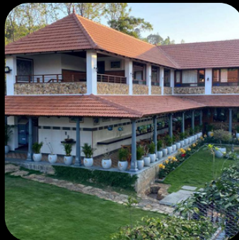
Mangalore Tile Roofing
